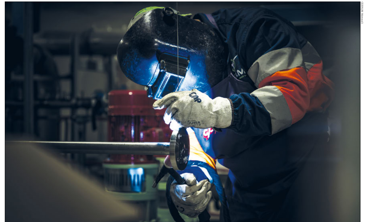
Skilled labour A technician at work in the new galleries of the High-Luminosity LHC. Trained people and upgraded suppliers are among the largest components of the machine's projected societal benefits.
