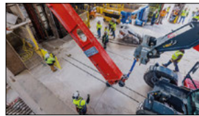
About 4500 tonnes of steel beams will be lowered to frame DUNE's detector modules.
