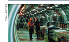
On the cover The 27-kilometre LEP tunnel, pictured in July 1991. 22
