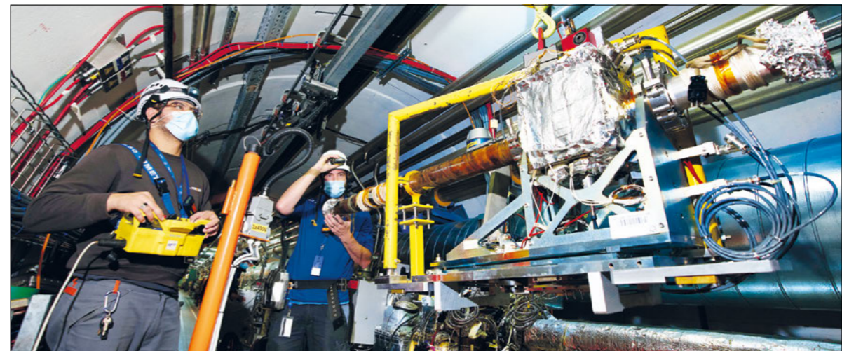
Heavy-ion collimation A crystal collimator is installed at the LHC, where it is used to deflect halo particles onto an absorber located roughly 90 metres downstream.
