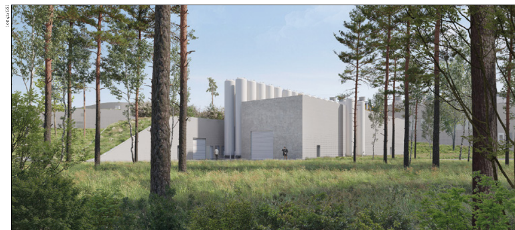
Blending in Artistic rendering of FAIR's cryogenics building upon completion, showing helium storage tanks (centre) and the nitrogen supply (right).
