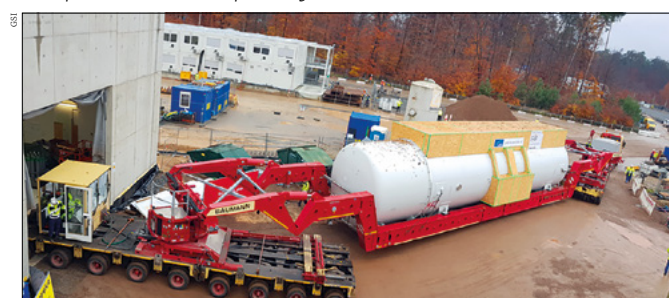
Heavy metal Transportation of the cold box into the front hall of FAIR's cryogenic supply building. Provided by Linde Kryotechnik, the cold box is 18 m long, 5 m in diameter and weighs 85 tons.
