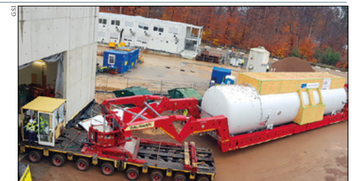
Special delivery Transportation of the cold box into FAIR's cryogenic supply building. 6
