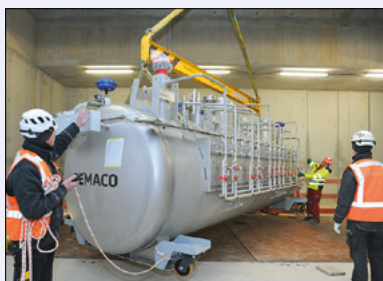
It's cold inside Installation of FAIR's cryogenic distribution system is proceeding at pace. Above: engineers oversee delivery of the central distribution box for provision of liquid helium to the SIS100 superconducting magnets.
