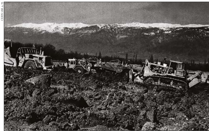
Excavation work for the North Experimental Area of the SPS began in April. In the photograph a bulldozer and two scrapers are in action, against the background of the Jura mountains, removing the top soil from an area of 8 hectares.
