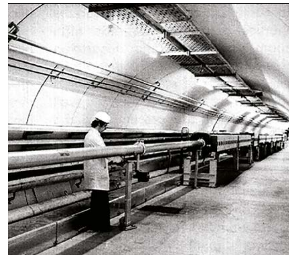
The vacuum chamber straddling a straight section of the 400 GeV synchrotron. A length of 970 m of the vacuum system has now been pumped down and is at 1 \times 10^{-8} torr. An ion pump can be seen hanging below the chamber at the centre of the straight section.
